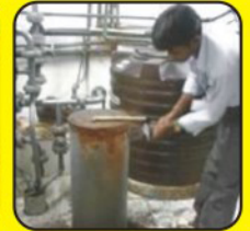
Removal of Rust
